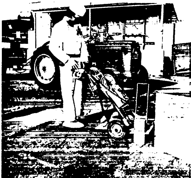
Fig. 42. Ground surface surveys with phoswicon detector.
