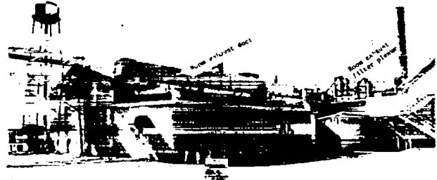
Fig. 16. Northwest side of Building 5.
