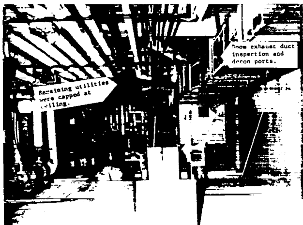
Fig. 11. Building 150 basement, overhead utilities.
